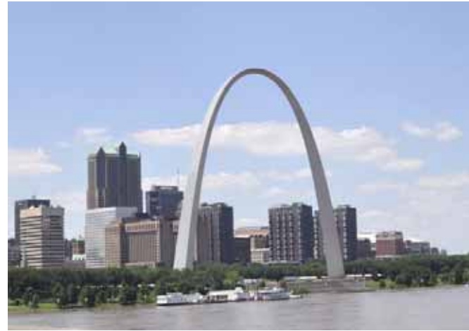
Expansion of the Gateway Arch Grounds to East St. Louis is proposed
